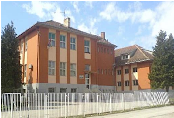
Figure 1. The school building used for energy performance analysis
